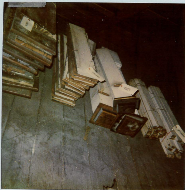
Treads, risers, newell posts and pickets in storage area in attic. All tagged.
