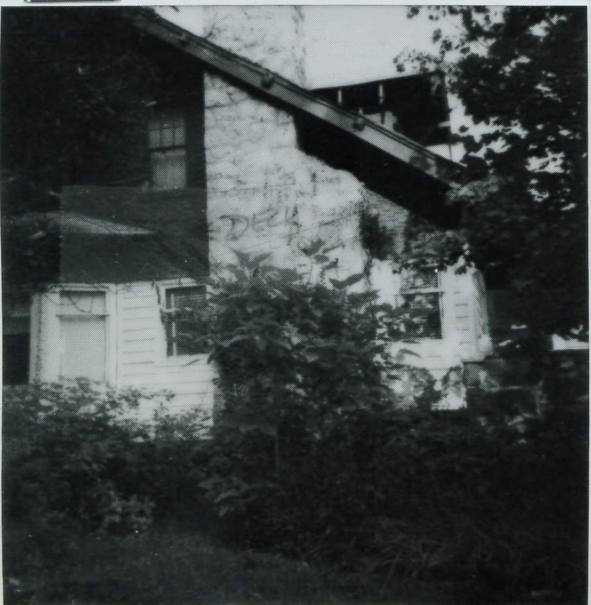
Side showing stairs + deck will be almost completely obscured from view (Before)
