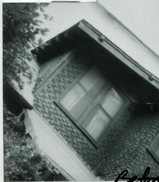
NOTE RAFTER ALL SAWED OFF / OTHERS ROTTED KNOTE roof line
