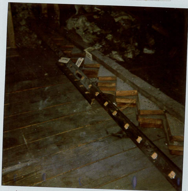
Handrails + stringers in place in attic. All tagged.
