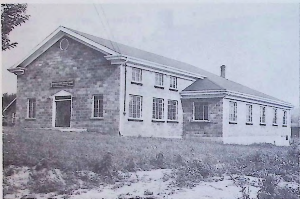
APPENDIX III NEW CINDER BLOCK CHURCH
