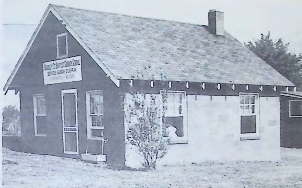
APPENDIX I CINDERBLOCK GARAGE BUILDING
